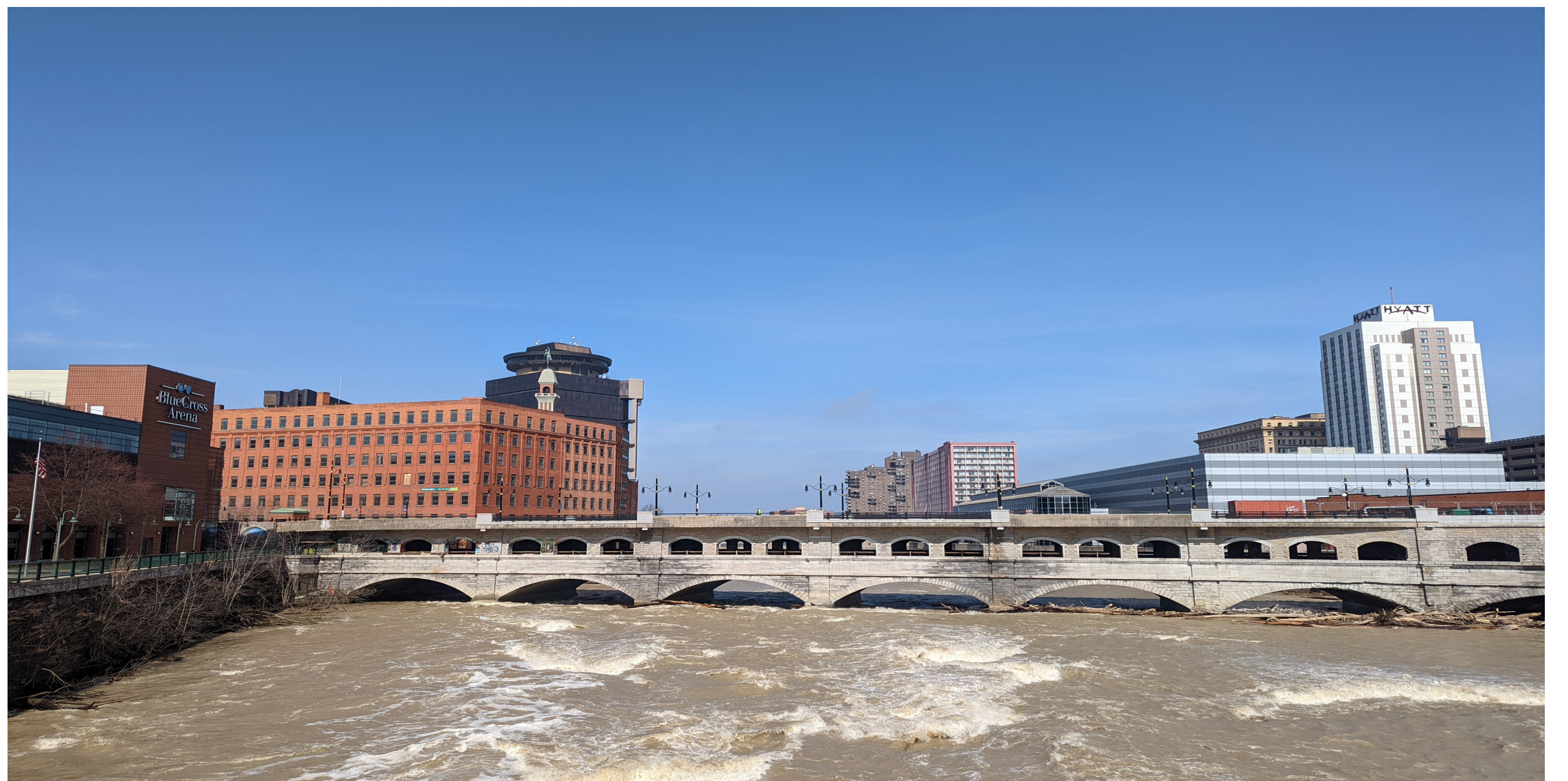
The Aqueduct from Court Street Bridge
