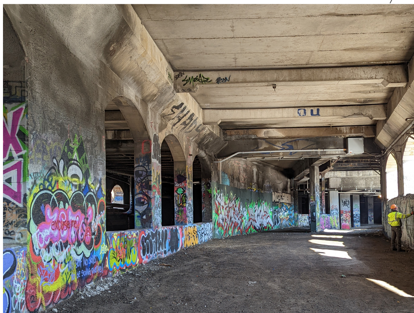
Subway Tunnel Looking East
