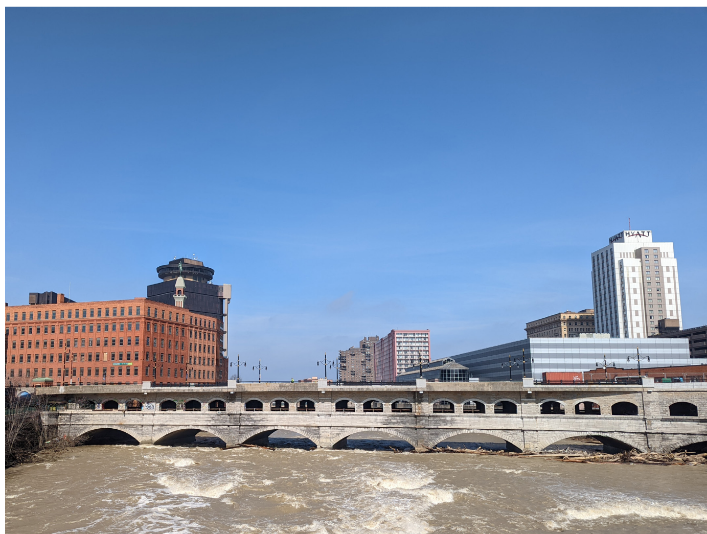
The Aqueduct from Court Street
