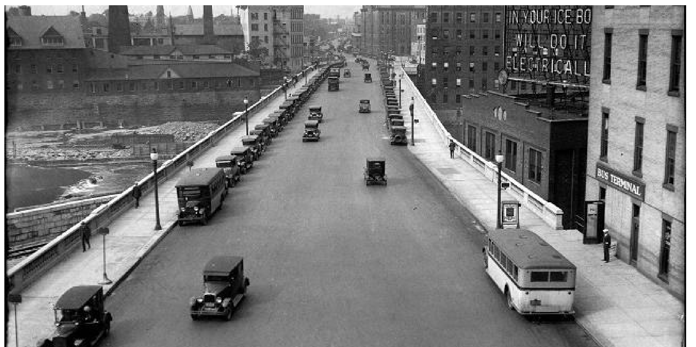
Broad Street Bridge (1925)
