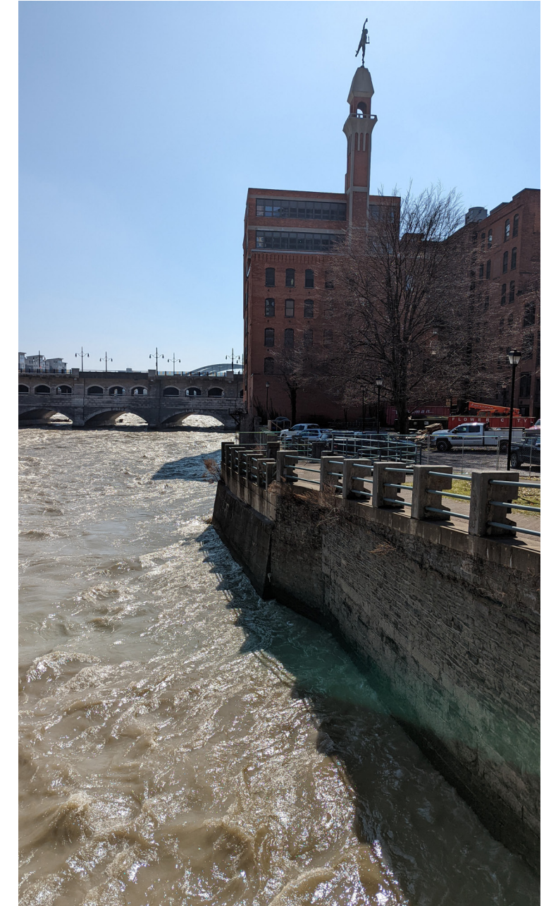
Aqueduct Building from Main Street Bridge
