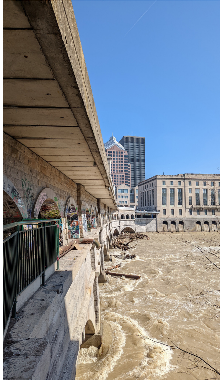
Aqueduct from War Memorial
