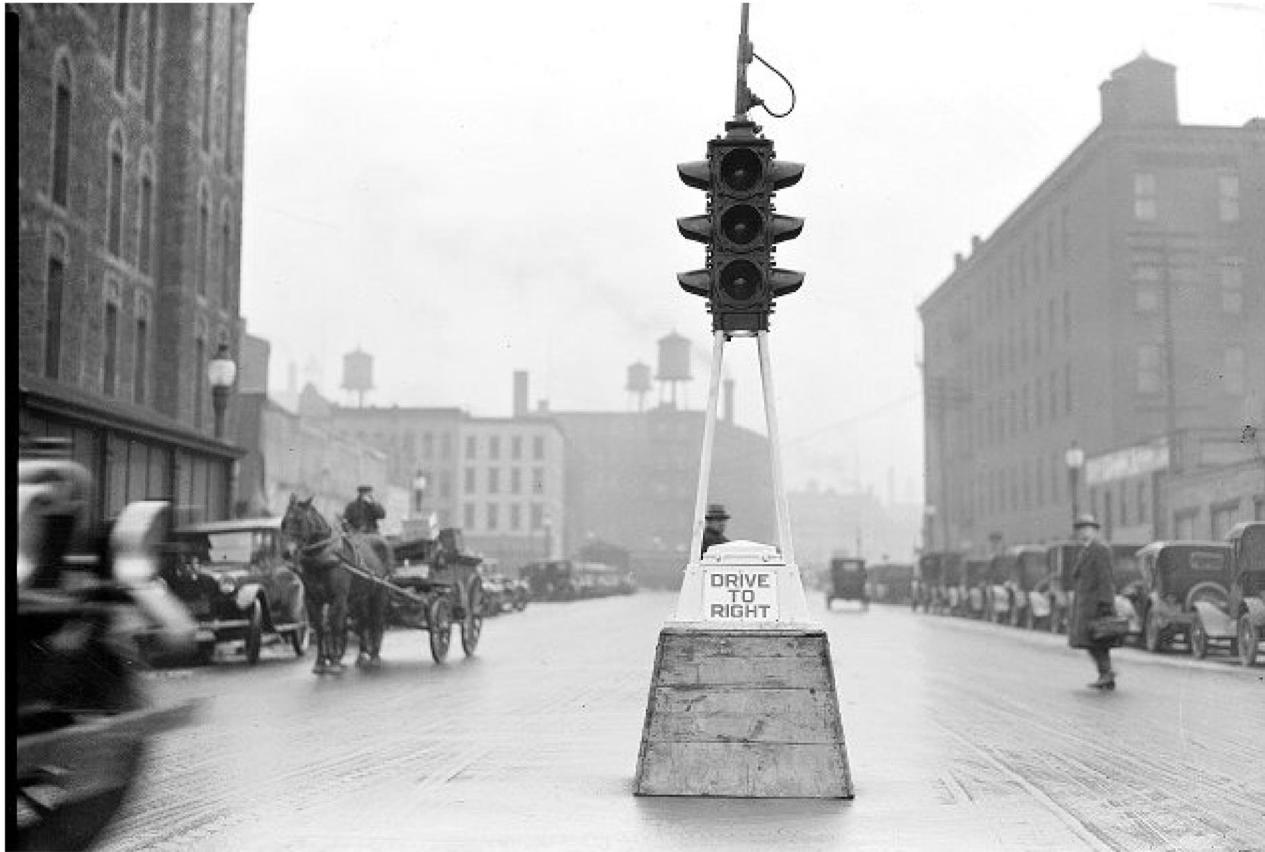
*This traffic signal of a type called the “silent policeman” or “silent cop” stands in the intersection of Fitzhugh and Broad Streets. The base is wooden. Just above the base is the sign “Drive to right”. Above that is a framework made of four wooden legs that supports a standard red-orange-green four-way traffic light. A horse-drawn wagon approaches the light. Automobiles are parked on both sides of the street.*
